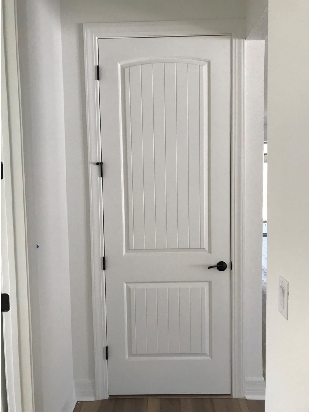
8' Cheyenne Interior Doors (Downstairs)
