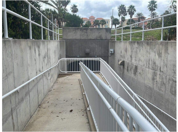
Tunnel to Beach Access
