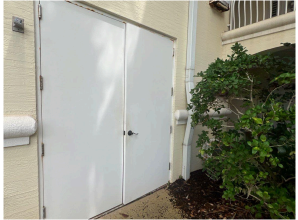
Typical Exterior Doors
