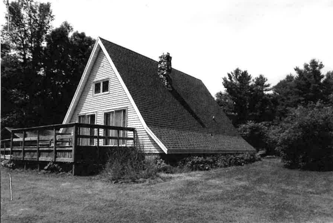
Photo One Caption view from the north 7-7-2022
