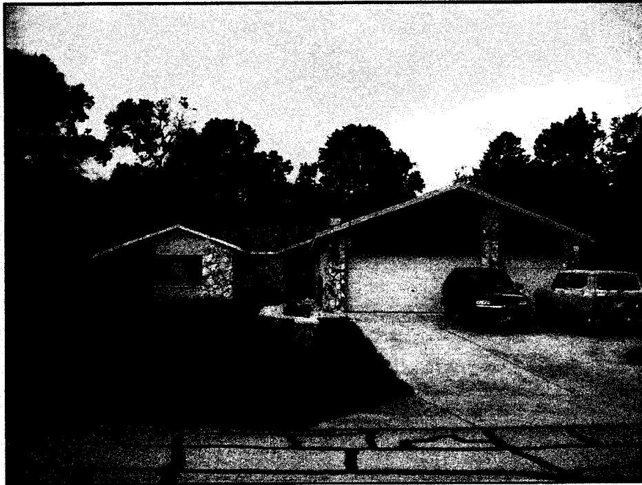
Photograph 1: The front of the house looking south.
