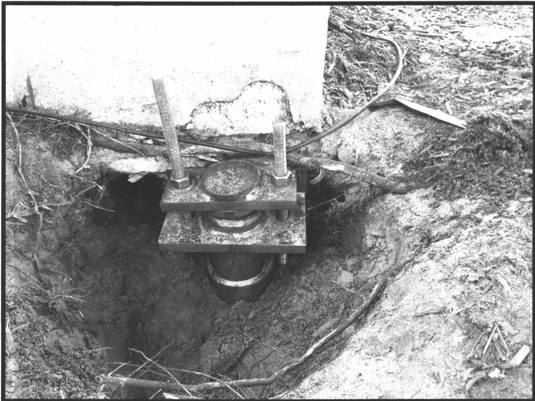
Photo 4: View of a typical completed pin and bracket.
