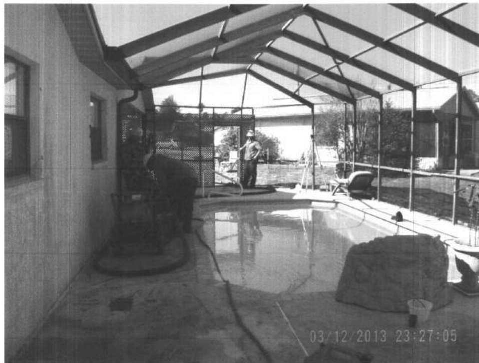
Picture 4: Rear elevation with grouting process on pool deck
