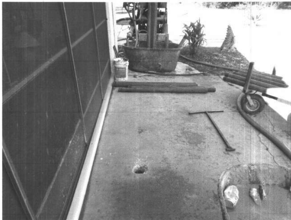
Picture 6: Core hole in driveway
