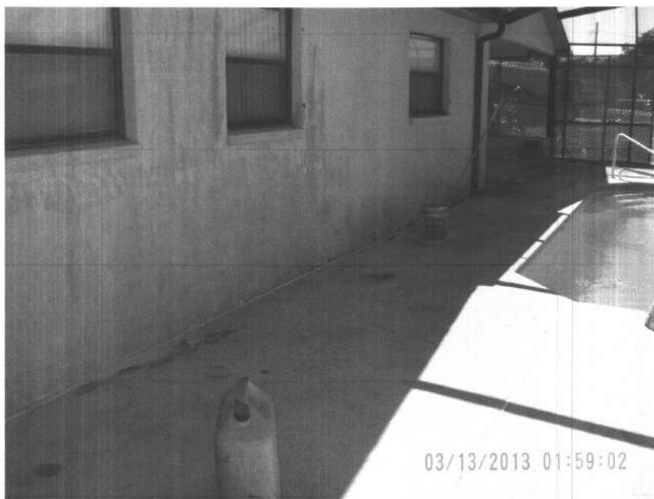
Picture 8: Filled core holes on pool deck
