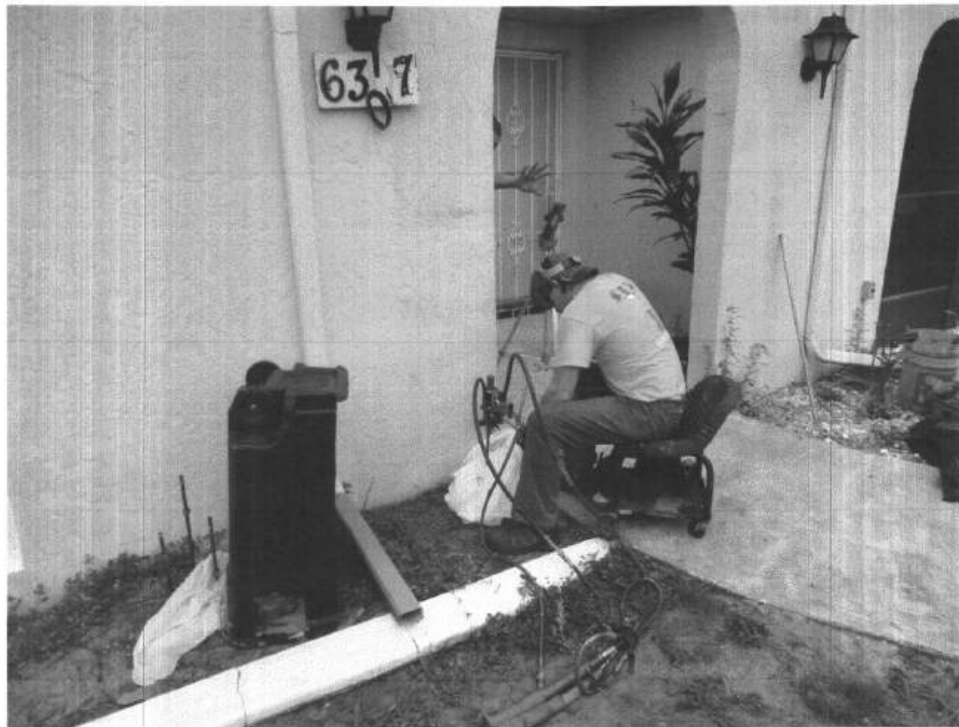
Picture 12: Pumping chemical injections
