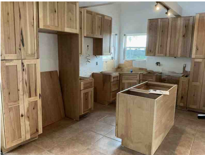
View of Kitchen
