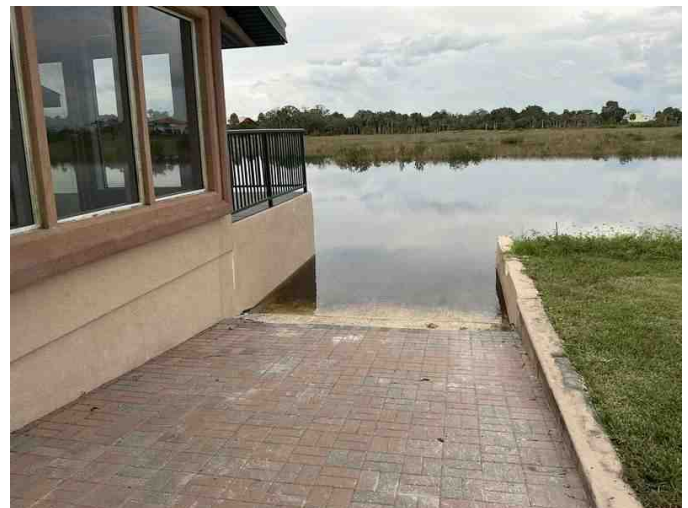
Additional Boat Ramp
