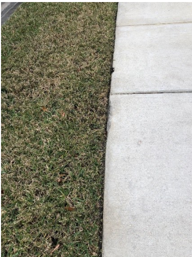
Example of Compliant Lawn Edging
