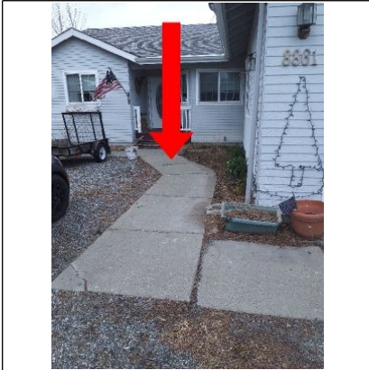
Recommend evaluation for repair of the deteriorating Concrete service walk leading from the garage to the porch located on the front of the home.
