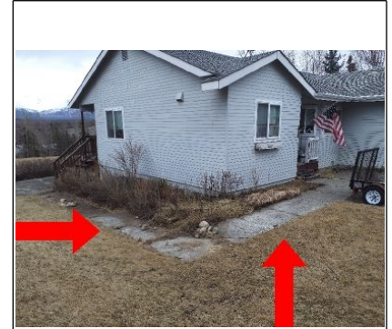
Photo of the concrete service walk located on the left-hand side home leading to the deck located on the back of the home.
