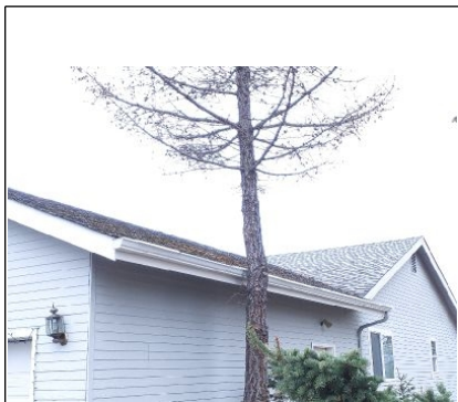
Overview of the roof.
