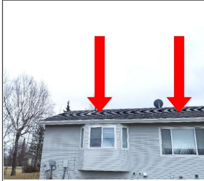
Recommend evaluation by a licensed roofing contractor for the removal of the moss growth occurring on the roof located on the right hand side of the garage and the backside of the roof.
