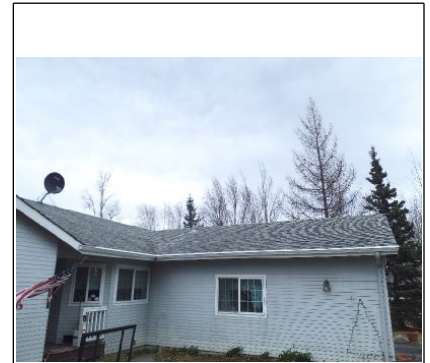
Recommend evaluation by a licensed roofing contractor for the removal of the moss growth occurring on the roof located on the right hand side of the garage and the backside of the roof.
