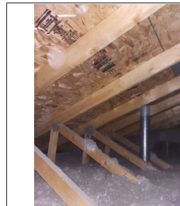
Overview of the attic.
