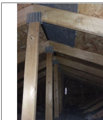
Overview of the attic.
