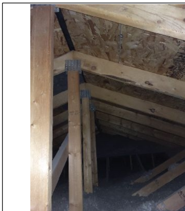
Overview of the attic.
