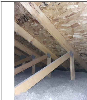
Overview of the attic.
