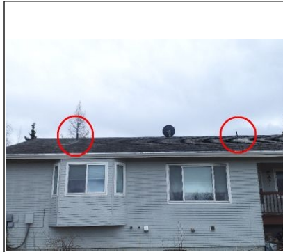
Photo of two Plumbing vents.
