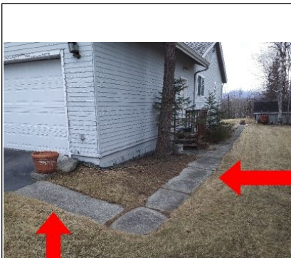
Recommend evaluation for repair of the deteriorating Concrete service walk leading from the garage to the porch located on the front of the home.
