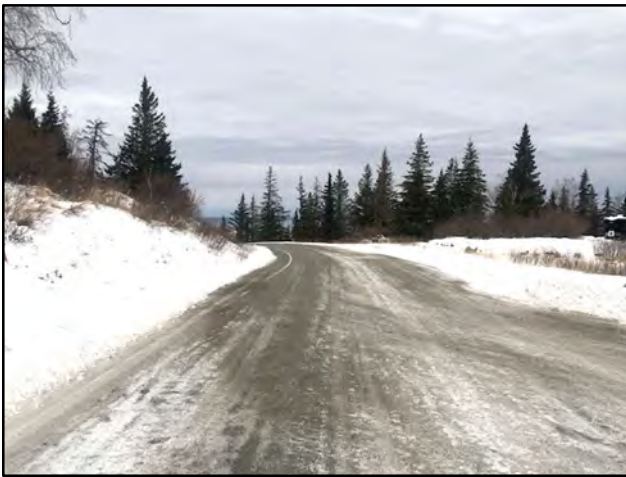
Westerly view on Potter Valley Road with Parcel 2 on left and Parcel 1 on right side of frame
