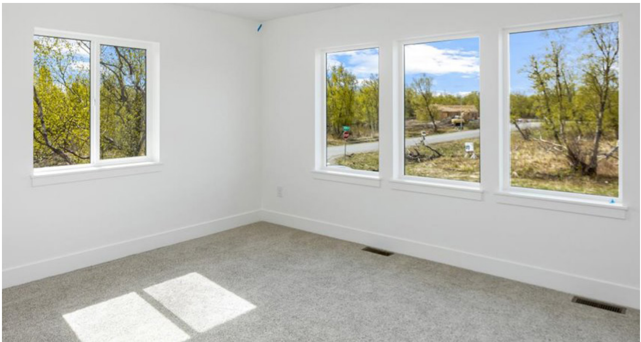
Upper Level Windows Square Edge, Sheetrock And Wood Sill
